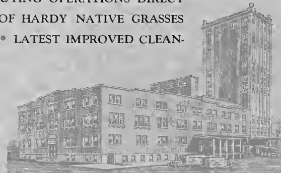
ASSEMBLING, CLEANING AND STORAGE PLANT ATCHISON, KANSAS
